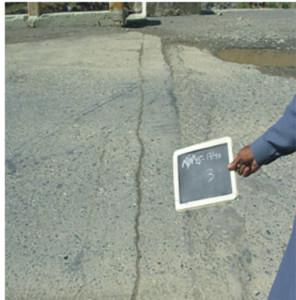
Fig. 8. Improperly repaired joint with bituminous material has cracked and restricted the movement
