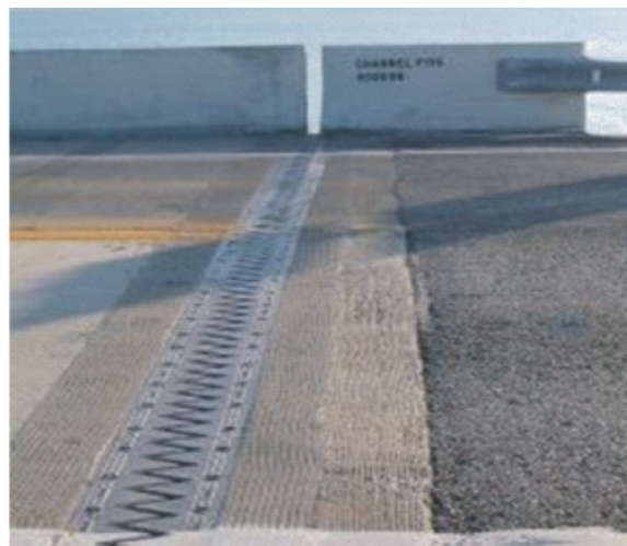
Fig. 1. View of the properly installed finger joint
