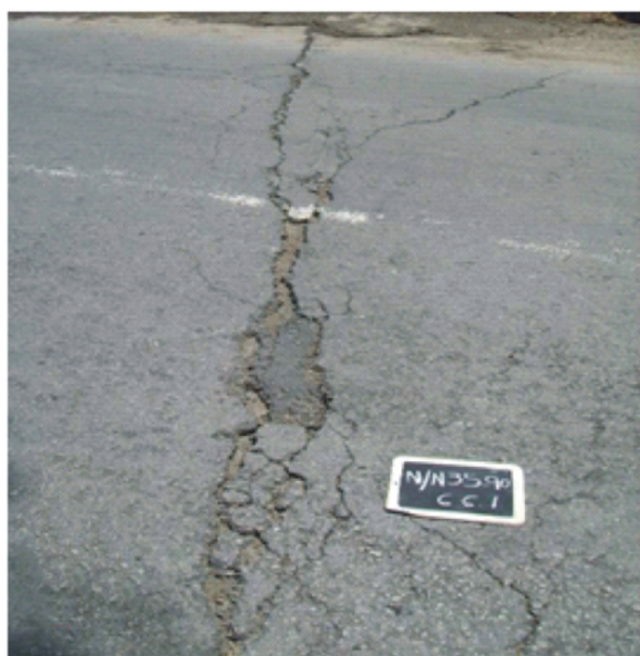
Fig. 3. Improperly repaired joint with bituminous material has cracked and restricted the movement
