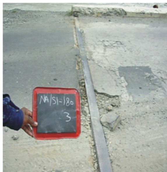
Fig. 4. Joint assembly is dislodged, causing noise and damage to the deck concrete
