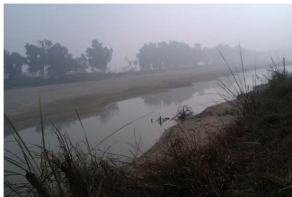
Fig. 3. Inadequate freeboard at 97.61 km of UJC
