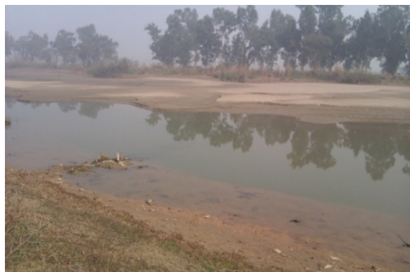
Fig. 1. Excessive silt deposition at 109.73 km of UJC
