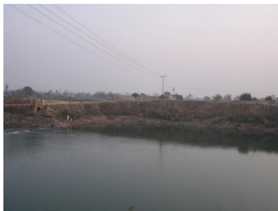
Fig. 2. Erosion of banks downstream at 99.02 km of UJC
