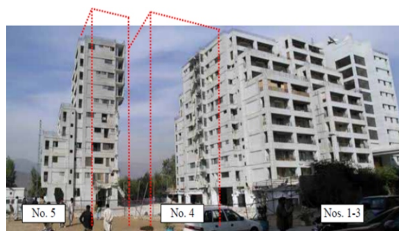
Fig. 1. The Collapsed Margalla Tower Islamabad Pakistan
