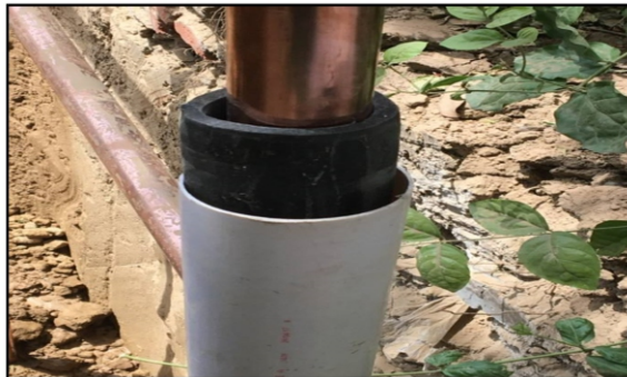
Figure 7: PVC Pipe Insulation over Rubber Insulation
