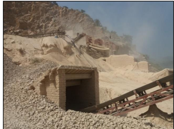
Fig. 1. Bazid Khel Crush Plant in Darra Adam Khel
