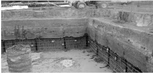
Fig. 13. Shoring System of Residential Building [2].
