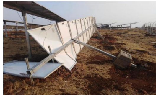
Fig. 23. Solar farm in Bhadla Rajasthan after wind storm [23].
