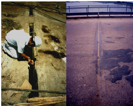
Fig. 18. Wide gap above pier P3 due to excessive settlement of the pier foundation (left), Status of the joint above pier number 3, 2001(right) [18].
