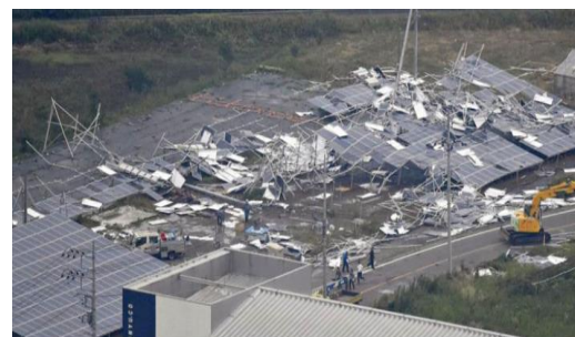
Fig. 24. Solar Farm in Gunma, Japan after wind storm [20].
