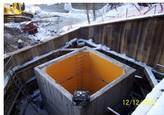
Fig. 12. Fox Hollow Sanitary Trunk Sewer Manhole London, Ontario [8].
