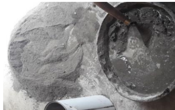
Fig. 6 Preparation of Mortar
